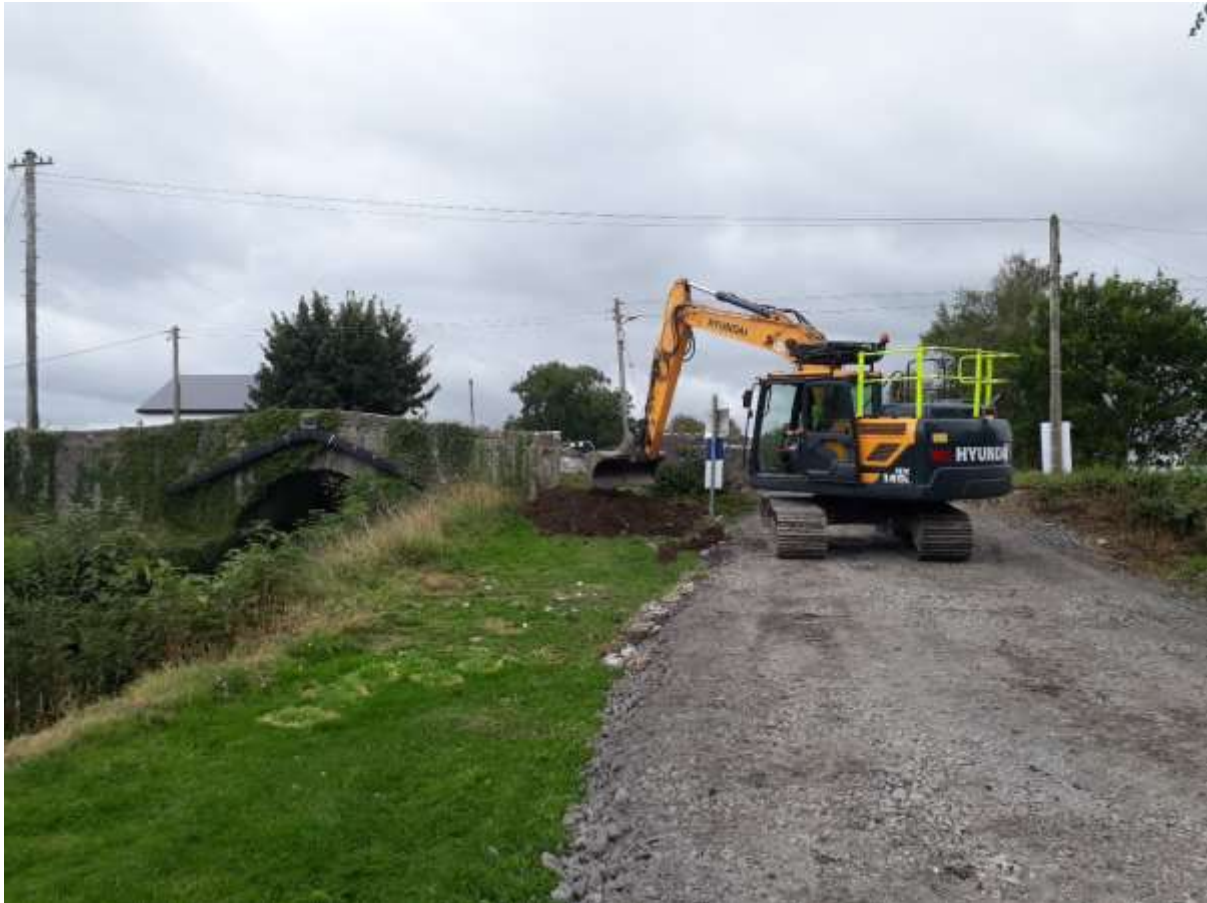
Fig 1 – CH13400 looking North to Spencer Bridge. Commencing works.
