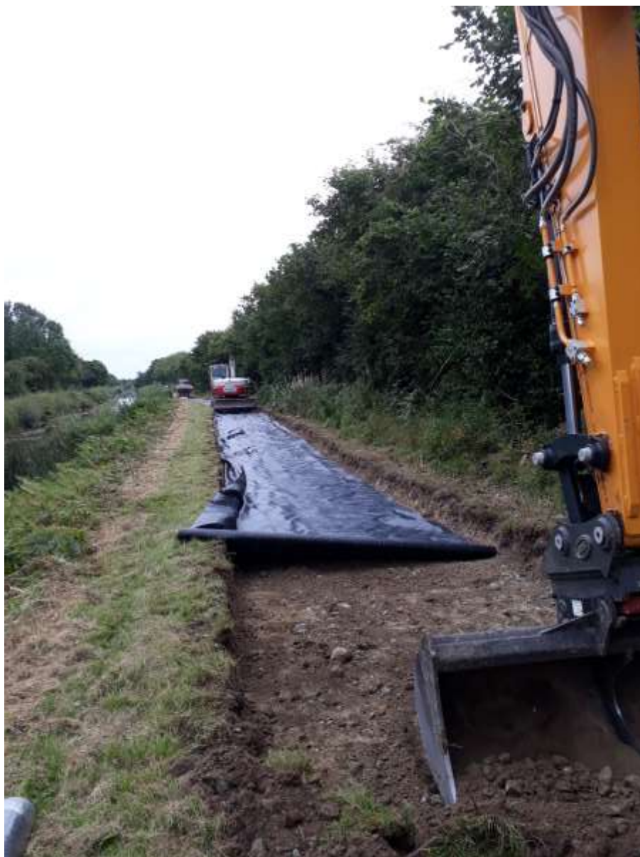
Fig2 – CH 28400 looking South to Fisherstown Bridge. Excavation & Terram layers
