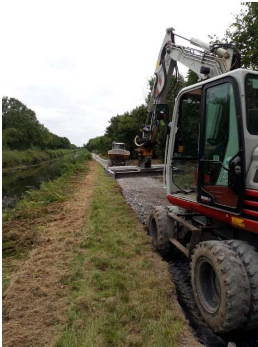
Fig 3 – Ch 27800 looking South – Stone installation
